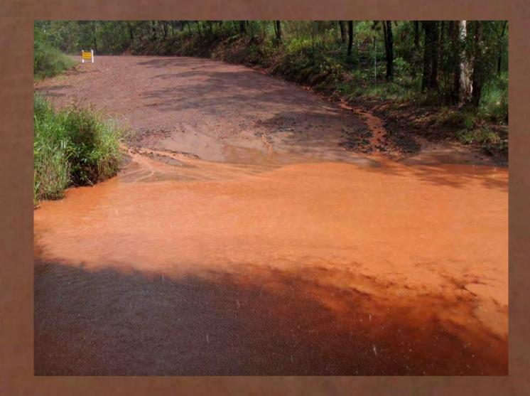
Sediment runoff from roads at stream crossings is a significant problem. Better road design and improved maintenance are urgently needed.
