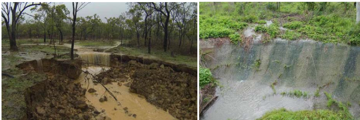
Plate 14 Young, rapidly advancing headcuts of alluvial gullies need to be stabilised with drop structures or rock grade control so that they do not develop into larger gullies and head scarps (Plate 1).
