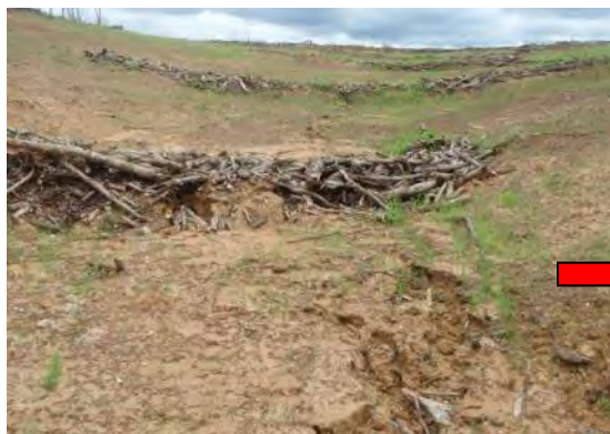
Headcut Re-initiation, Jan-2012
