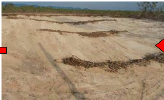
Diverting Hillslope Water, Adding Wood Weirs, Dec-2011
